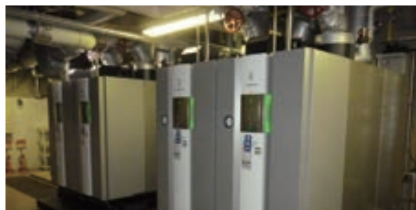
Installation of highly-efficient boilers in the Injection Building (Shizuoka site)
