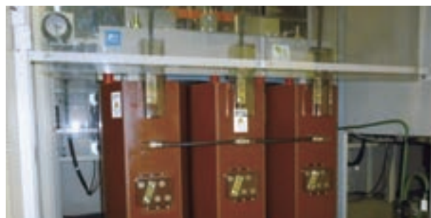
Installation of molded transformers in the Oral Solid Formulation Building (Shizuoka site)
